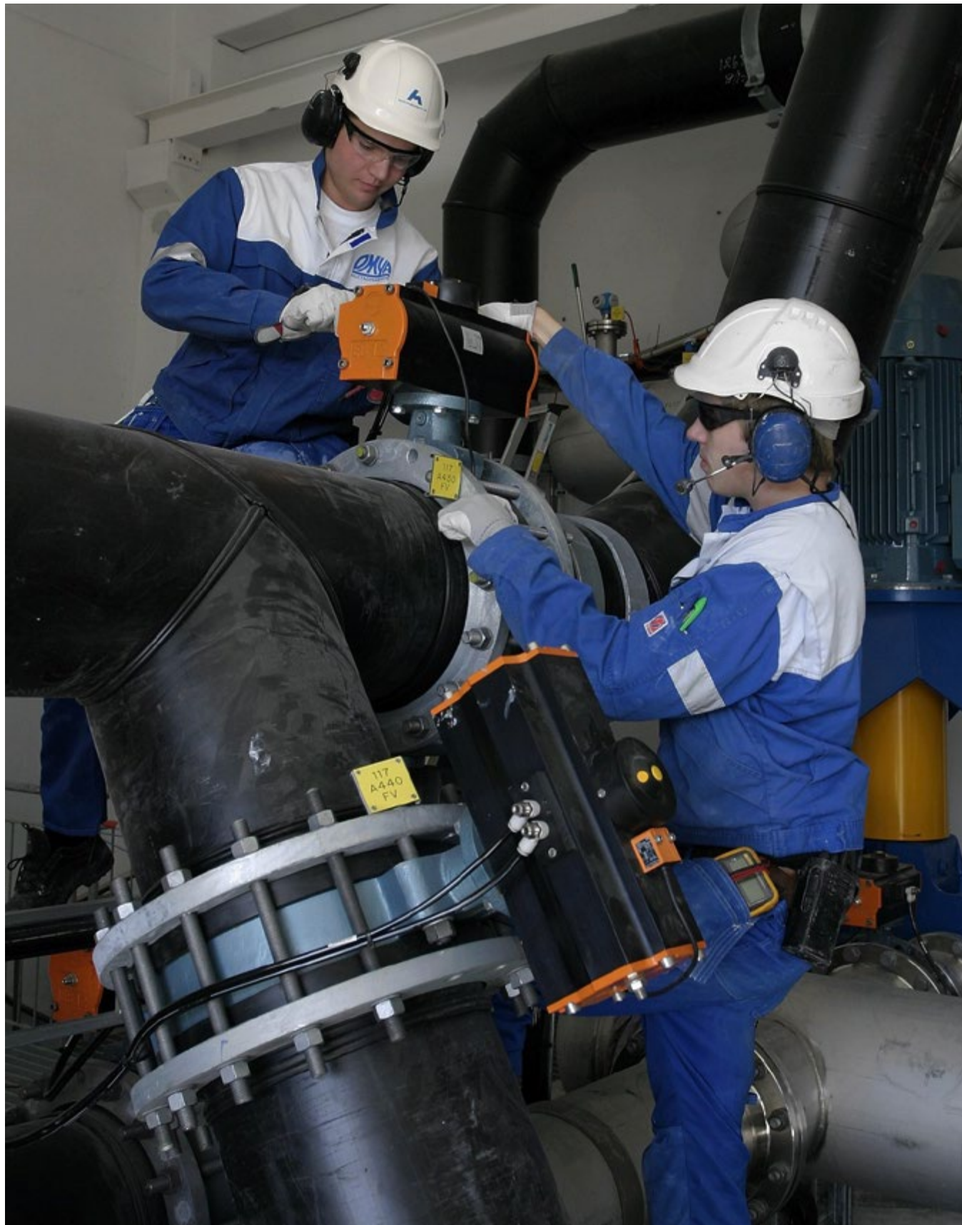
Mounting a control valve in a cooling circuit. The work is being carried out by apprentices at Hustadmarmor AS. Photo: Hustadmarmor A/S
